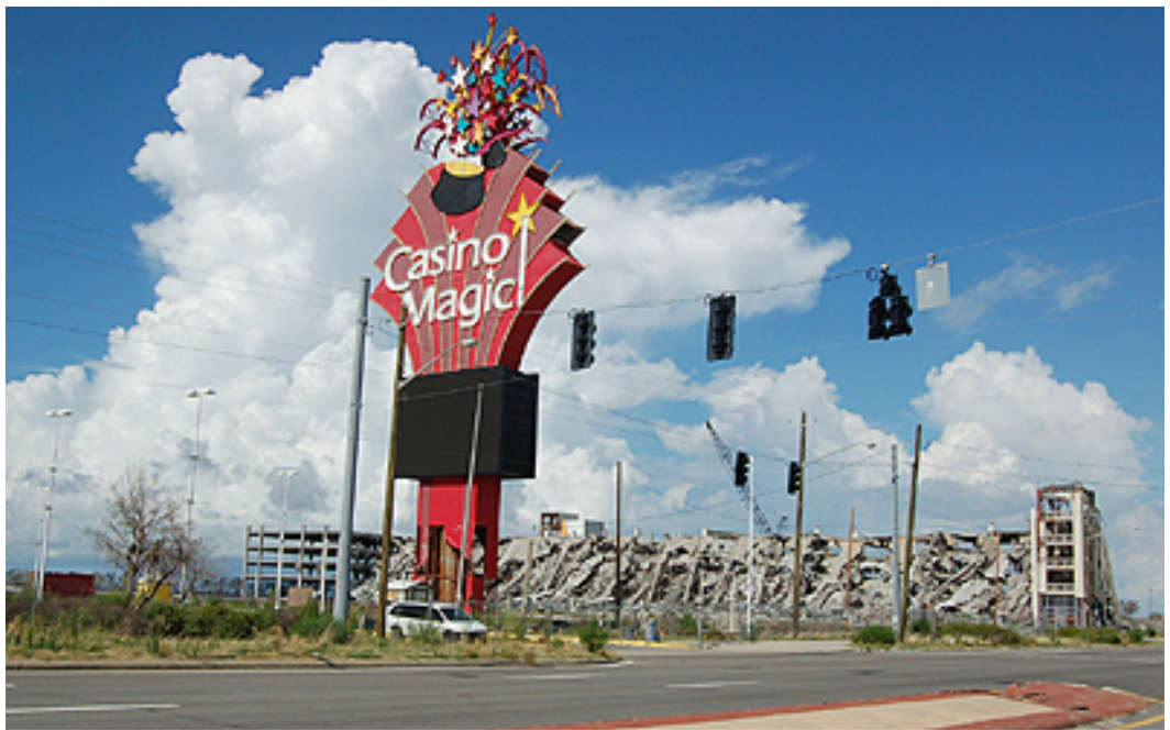
Gulf Coast casino and rubble
