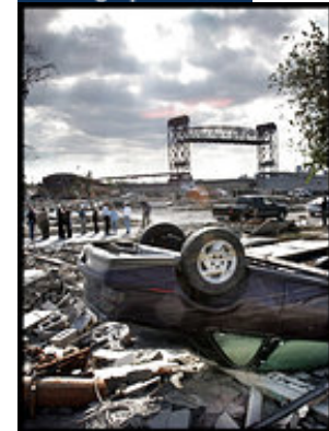
New Orleans's 9th Ward was largely destroyed when levees broke after Hurricane Katrina, and the infrastructure must be repaired or replaced. Rebuilding the levees alone is expected to cost at least $20 billion. (By Robert F. Bukaty -- Associated Press)
