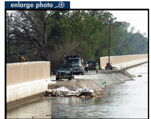
Workers repair a section of the levee at the 17th Street Canal, which breached and caused flooding. (By Ricky Carioti -- The Washington Post)
